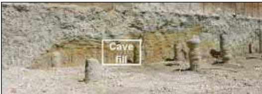
Day 3-Figure 11. Filled in cave in the Dammam Formation as seen in a construction site in Doha (Duggan, 2014).
